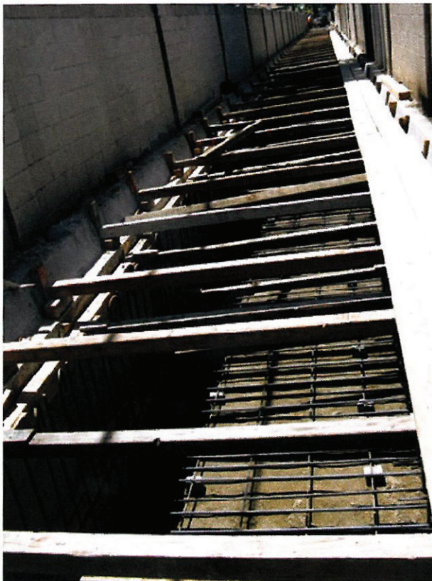
Thornton/Brady Box Channel Under Construction
