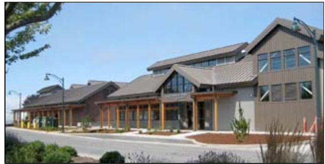
Photo courtesy of Harris & Associates [enlarge] The 25,000-square-foot Lighthouse Point Water Reclamation Facility is designed to treat a peak flow of 3.1 million gallons per day.
